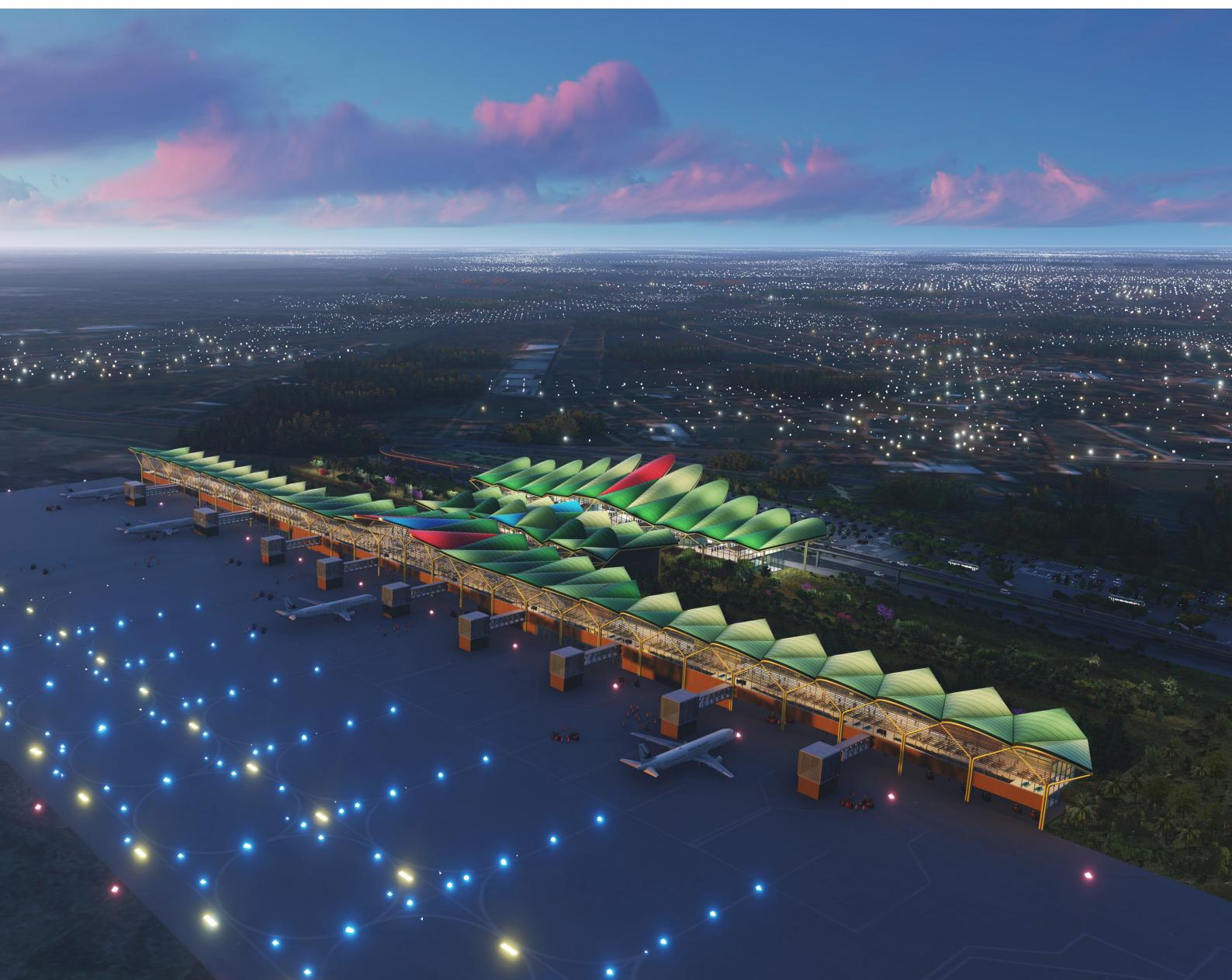
The New Terminal Building (NTB) at Silvio Pettrossi International Airport is made up of a large volume on the airside and another one on the landside. However, this second piece, of mixed use, is divided as well into two pieces, separated by green patios that introduce natural light inside the building and provide passengers and users with views to the outside through fully glazed façade of a light appearance.
