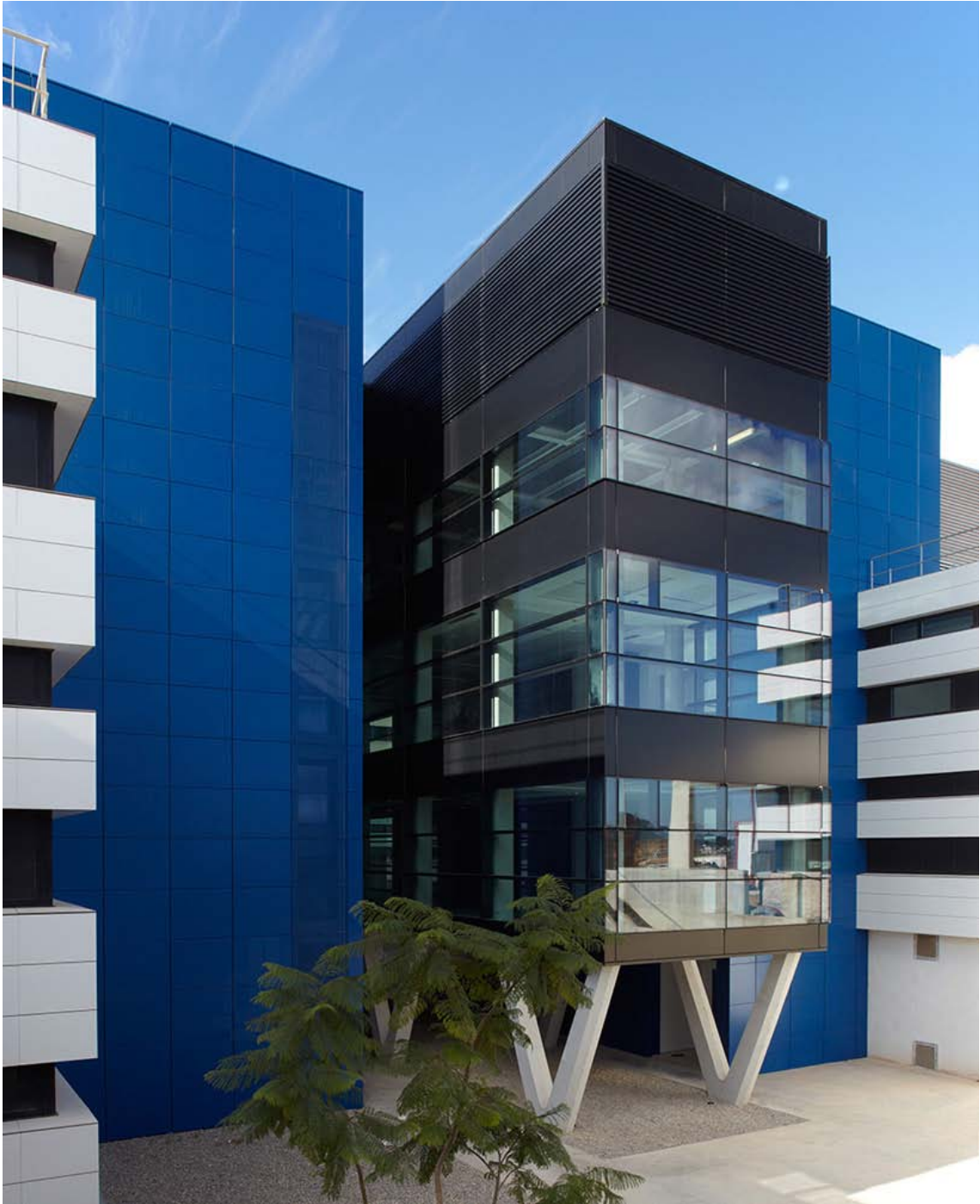
exterior with raised structure
